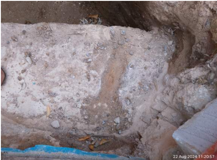
02 - EX FND AT ACCESS WAY - EMBEDDED SHUTTER - BUT OTHERWISE AS 01
